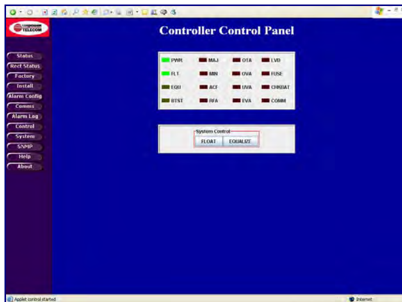
Figure 16 - Controller Control Panel WEB Page (typical)
